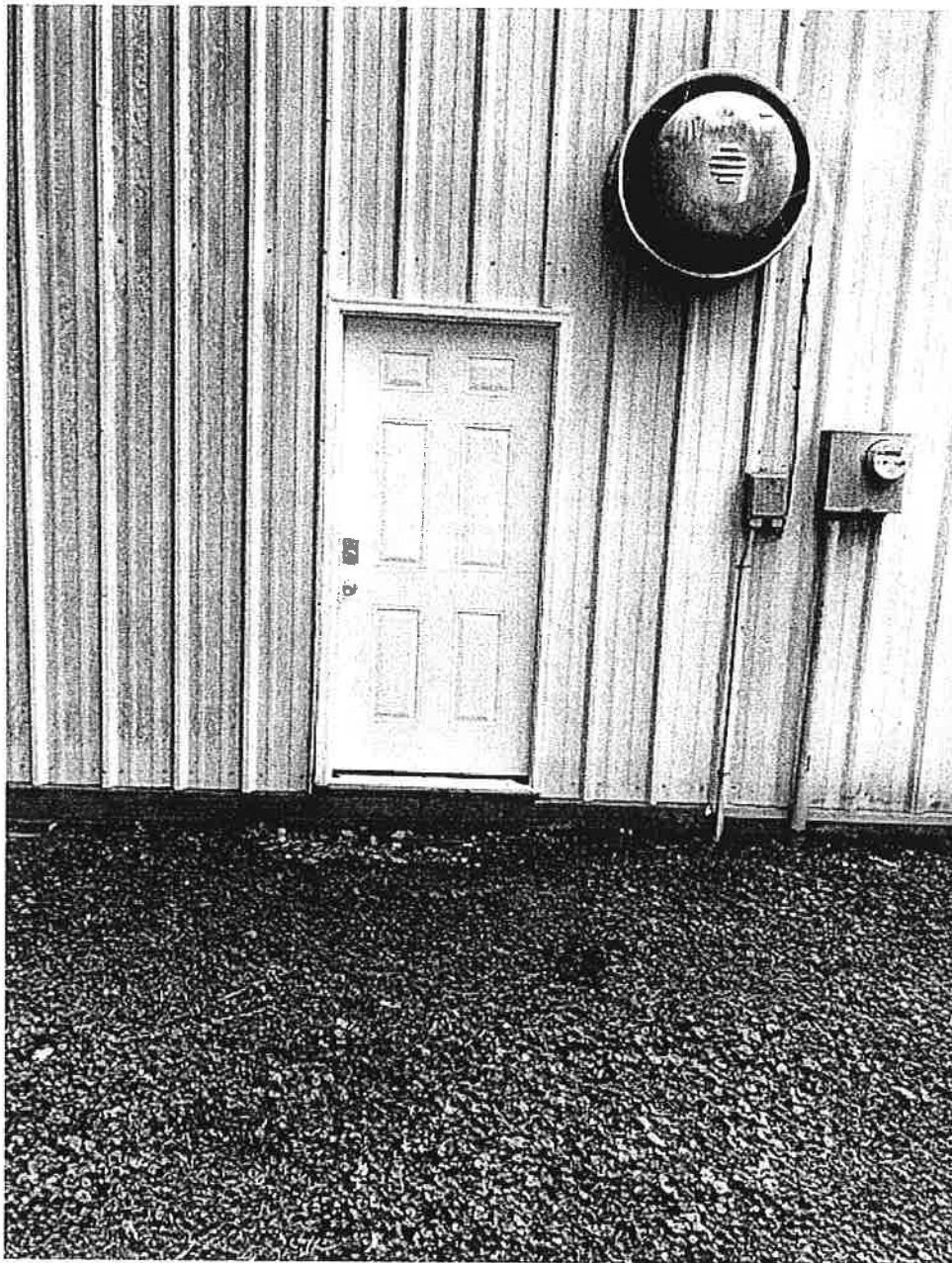
Main entrance to fire department. Needs APO sign.
