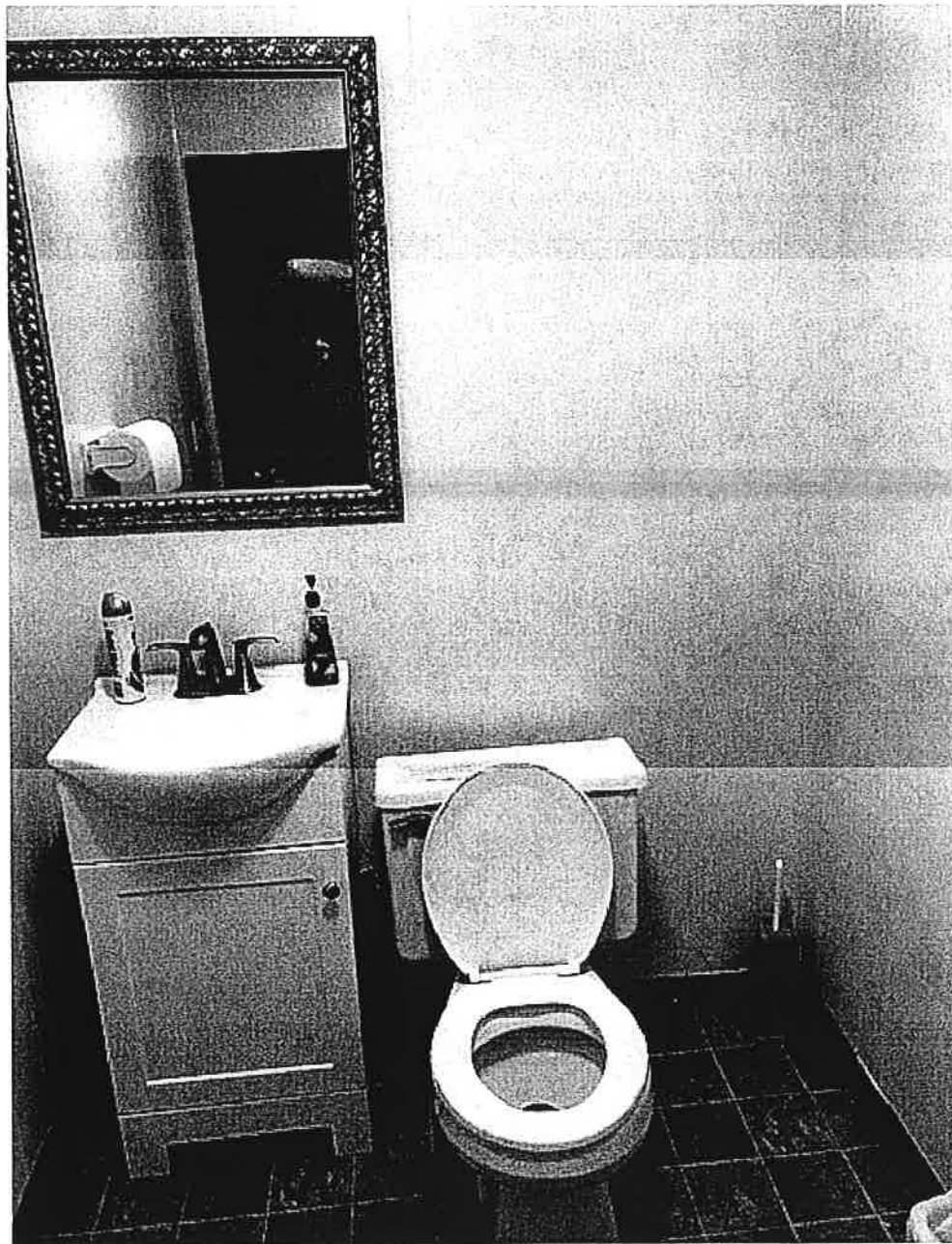
Women accessible toilet room with toilet, lavatory, and hand towels
