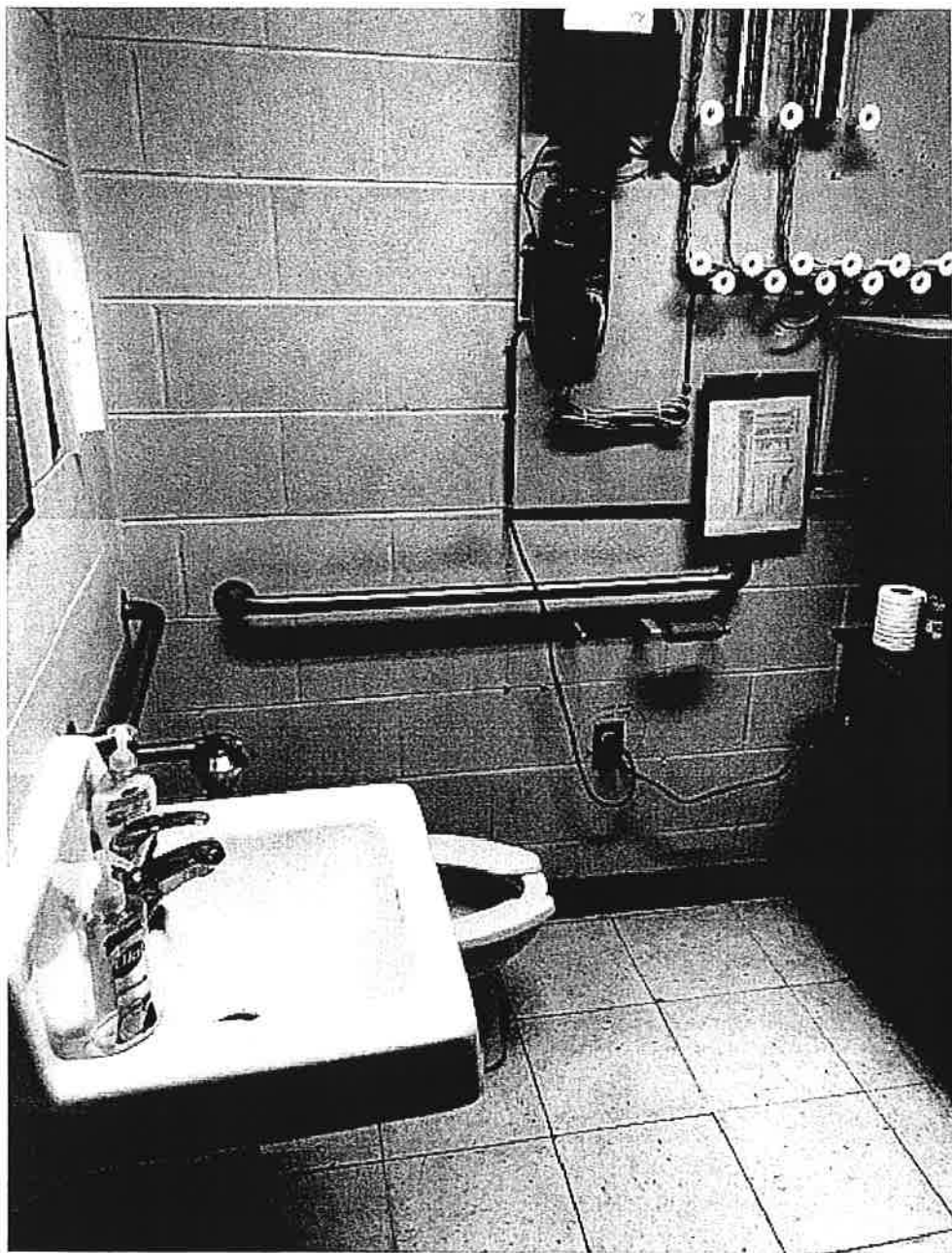
The toilet room in the Reception office
